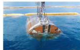
海中からの掘進機の回収 Collecting a tunneling machine from the ocean
