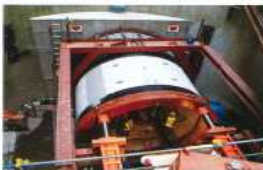
超大口径管の推進状況(発進立坑) The jacking method for the ultra-large diameter pipes is in process (starting shaft)
