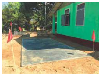
<Foundation for Pre-filtration and Filtration unit>
