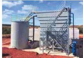
【Cambodia】 Water Treatment Plant in Modulkiri Province
