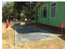
<Foundation for Pre-filtration and Filtration units>
