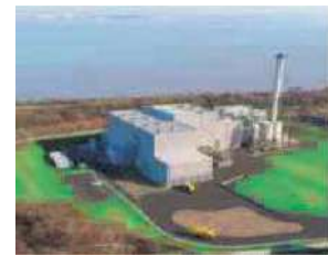
【UK】 WtE Plant for Hooton Bio Power
