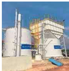
【Myanmar】 Water Treatment Plant in Thilawa SEZ
