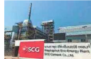
【Thailand】 WtE Plant for SCG in the Industrial Park, Rayong
