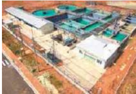
【Vietnam】 Centralized Wastewater Treatment Plant in the Long Duc Industrial Park
