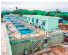
【Vietnam】 Water Treatment Plant in Thai Nguyen Province
