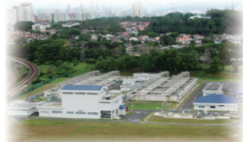
Sewage Treatment Systems
