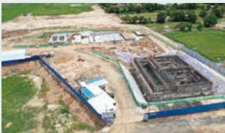
Water supply system expansion project in Kampong Thom, Cambodia
