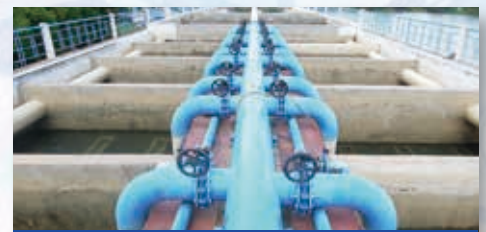
Water treatment plant for technical cooperation
