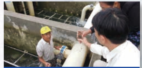
Preliminary survey and confirmation of filter sand
